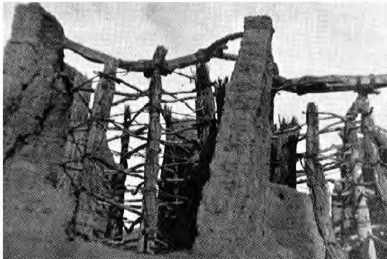
Vestiges of a vertical panemone wind mill at Seistan, Iran. The rotors were made from fabric or bundles of reeds and wood.
