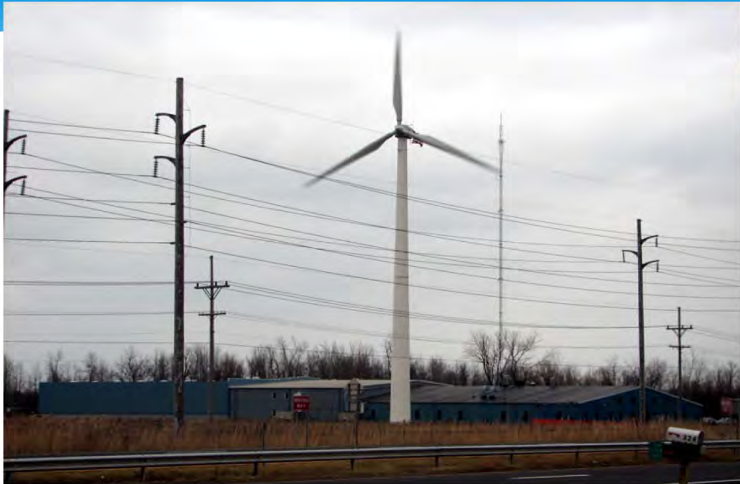
Single wind turbine providing power to a small business at Rochester, New York: Harbeck Plastics, Inc. Its surplus production can be wheeled into the electrical grid. Photographs courtesy: Chris Kabureck.
