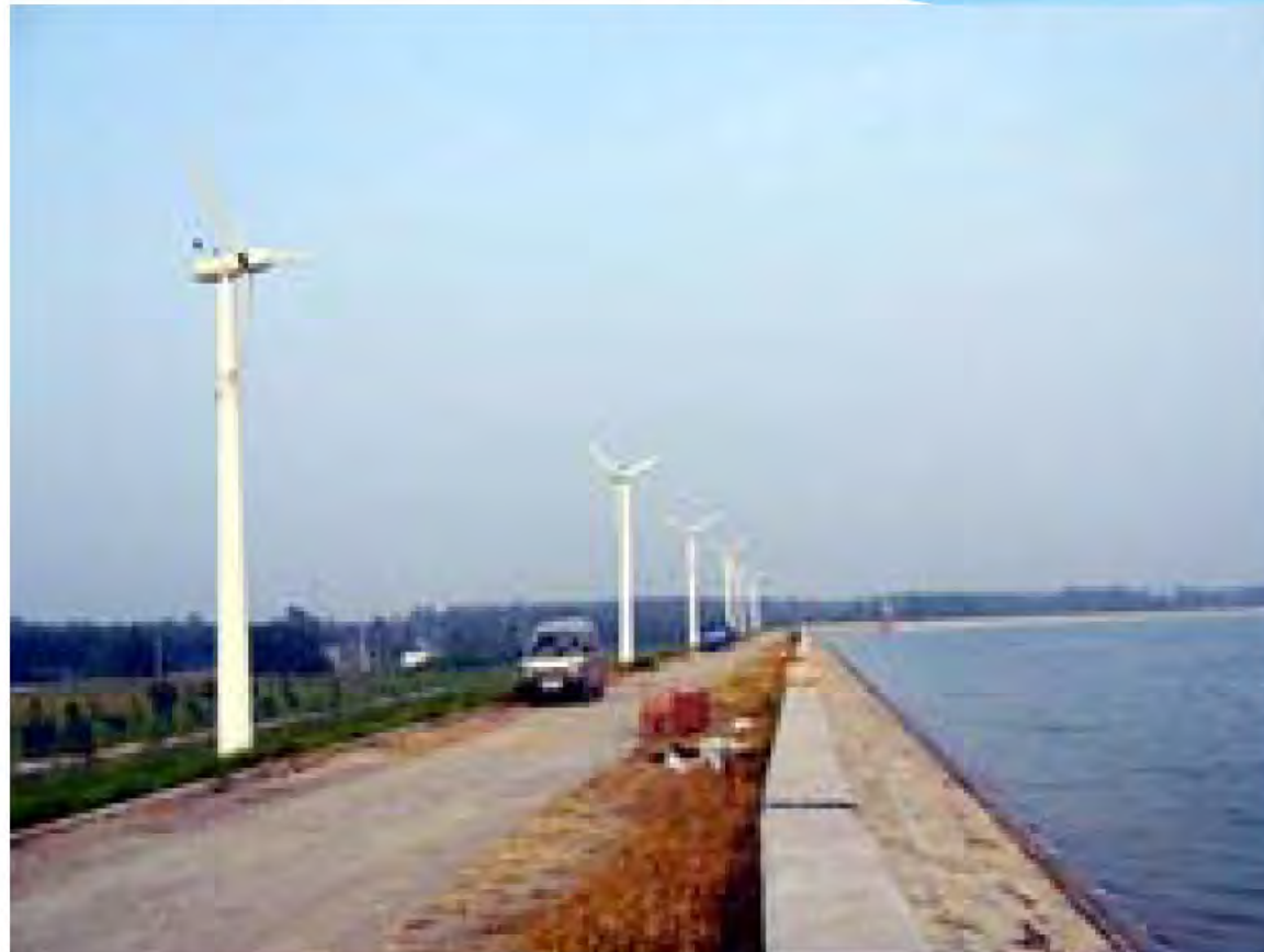
Row of HGenerators 3.4 kW turbines along water shore.
