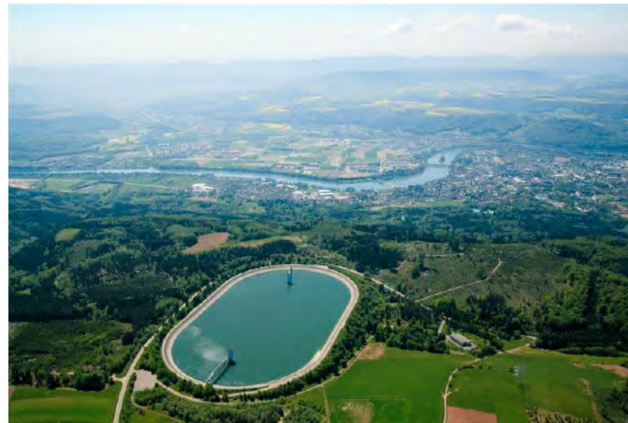
Eggberg reservoir supplies water to the Schluchsee power plant. Schluchseewerk AG Photo.
