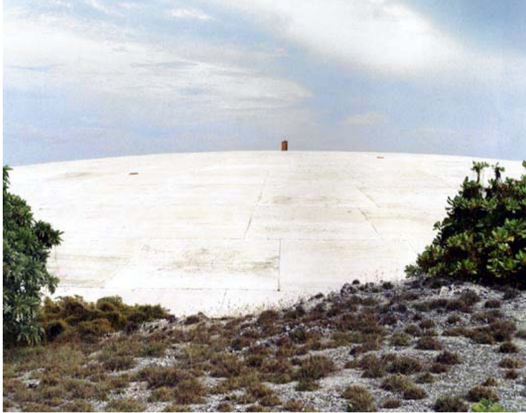
Figure 20. Concrete dome 18 inches in thickness entombs 111,000 cubic yards of contaminated soil and debris on Runit Island. As a prank, a red painted barrel on its top makes it visible as a nipple from aircraft flying overhead.
