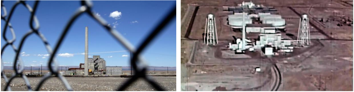
Figure 11. Views of the Hanford piles rising 120 feet above the desert floor with the water cooling treatment facilities, and the Columbia River in the background.
