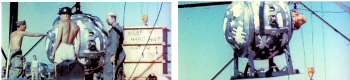
Figure 33. Trinity device before installation of initiators.
