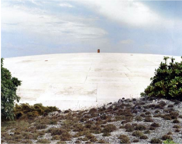
Figure 65. Concrete dome 18 inches in thickness entombs 111,000 cubic yards of contaminated soil and debris on Runit Island. As a prank by bored service-personnel, a red painted barrel on its top makes it visible as a nipple from aircraft flying overhead.
