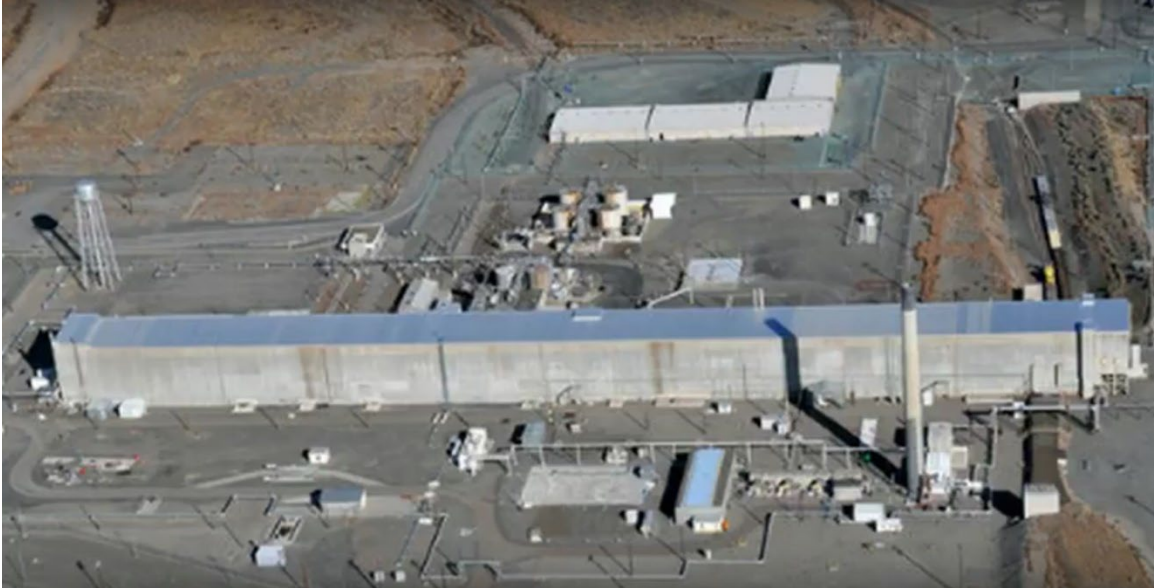
Figure 37. Exterior of Purex reprocessing canyon showing access through covered tunnels at the right hand side. Fuel from reactors was brought in in underground tunnels in railroad cars at the right side. There are two tunnels: One is approximately 360 feet long and the other is approximately 1,700 feet long.
