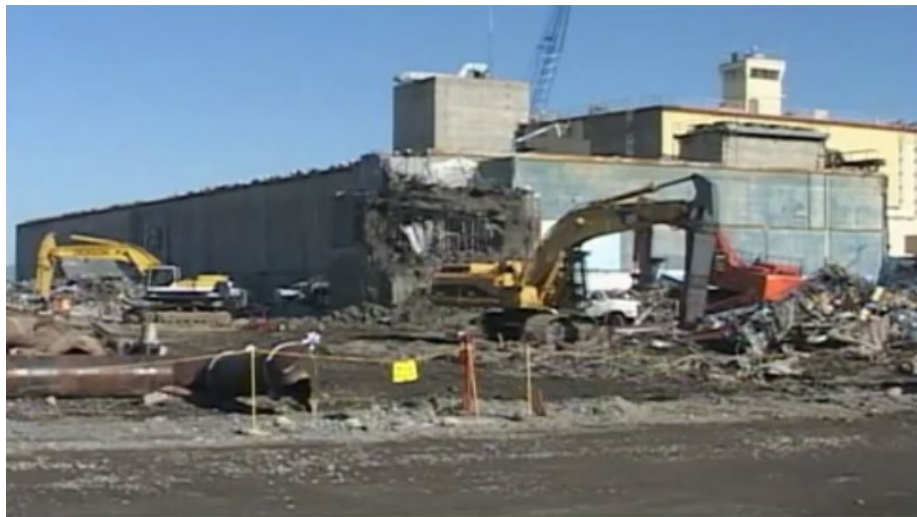
Figure 48. Removal and burial of contaminated structures at Hanford.
