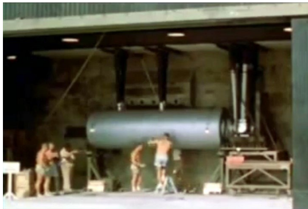
Figure 16. Exterior of the Castle Bravo device using lithium deuteride.
