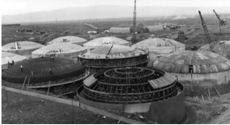
Figure 45. Double-walled high level waste tank farm at the Hanford reservation site, Washington, USA.
