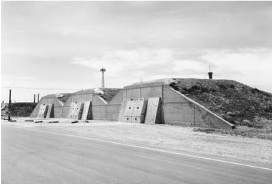
Figure 24. Nuclear weapons staging bunkers or igloos.
