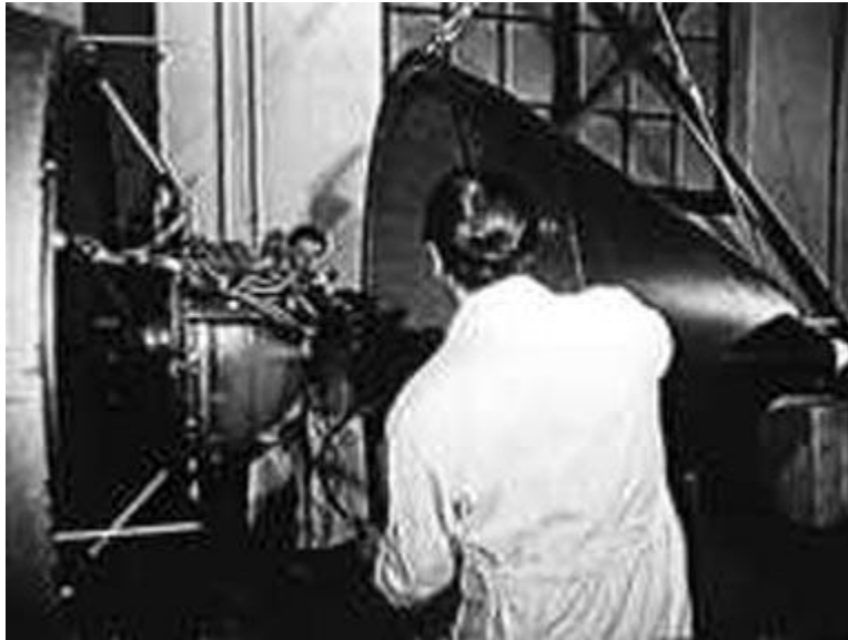
Figure 22. Assembly of the 100 Mt of TNT equivalent Russian device, Tsar Bomba. Its yield was intentionally reduced to 57 Mt by reducing the fusion charge and possibly using a lead damper instead of U^{238} in the third stage.
