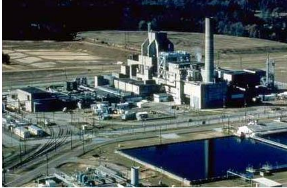
Figure 13. The Savannah River Heavy Water Reactor for the production of tritium from highly enriched U^{235} naval reactors fuel in LiAl alloy.
