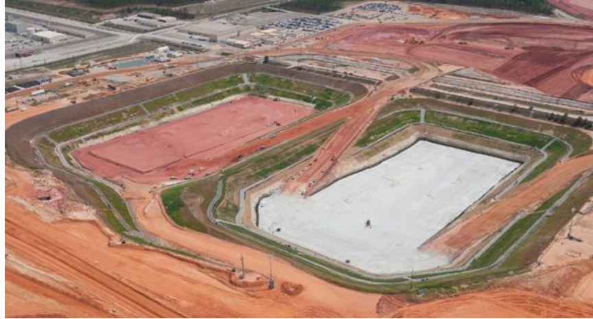
Figure 18. Foundations for the Vogtle units 3 and 4. Source: Southern Nuclear Company.
