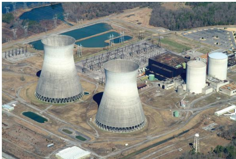
Figure 11. Tennessee Valley Authority, TVA Bellefonte Unit 1. Source: TVA
