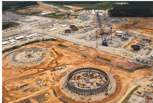
Figure 1. Georgia Power Vogtle plants units 3 and 4 under construction, 2013.
