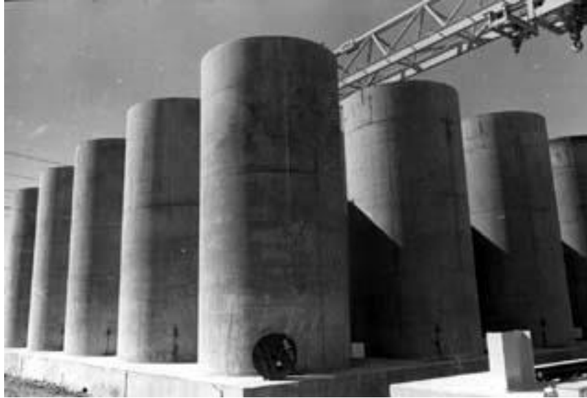
Figure 10. Onsite storage of Spent Nuclear Fuel in concrete silos at reactors sites.
