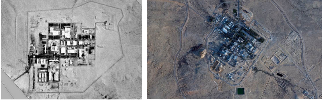
Figure 34. Nuclear Research Facility (NRF) Dimona Heavy water, natural uranium, 120-150 MWth plutonium and tritium production reactor, Negev Desert.
