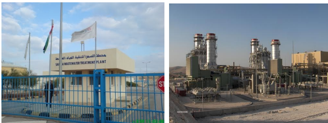
Figure 44. Khirbat Al Samra waste water treatment plant and gas turbines power plant near Balama, 40 km from Amman, Jordan.
