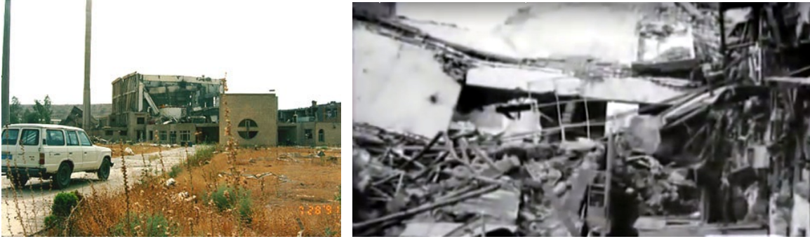
Figure 14. Osiraq, Tamuz building destroyed by the Israeli bombing raid, Operation Opera, June 7, 1981, Iraq.
