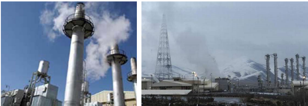
Figure 27. Heavy Water plant distillation towers at Arak, IRI.
