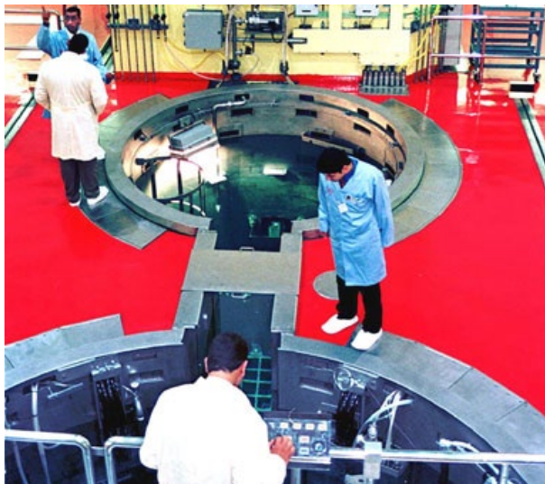
Figure 20. Interior views of the ETRR-2, open pool type 22 MWth research reactor at Inshass, Egypt.
