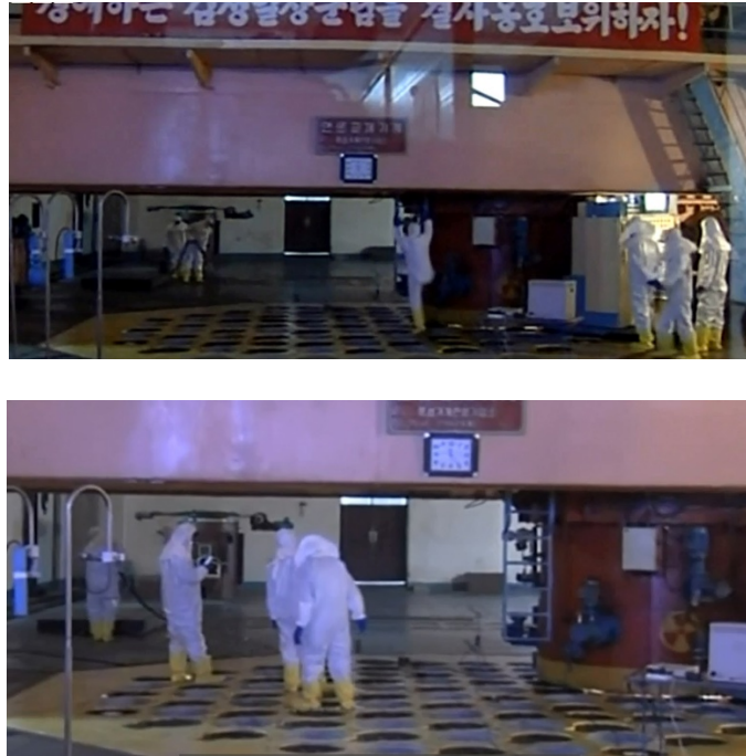
Figure 5. Inside view of Yongbyon-1, 5 MWth graphite-moderated, gas-cooled research reactor in the DPRK in a May 1992, IAEA Photograph (top).
