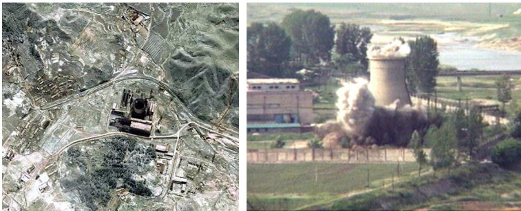
Figure 8. Aerial photograph of the Taechon 200 MWe power reactor under construction and the Yongbyon 1, 5 MWth research reactor in the DPRK. The cooling tower that appears to have been demolished in 2008 as a result of agreements was reconstructed in 2013.
