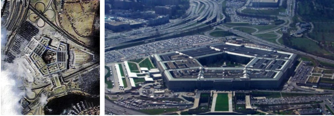
Figure 65. A one-meter resolution photograph taken by the Ikonos satellite showing a wing under reconstruction at the Pentagon building.
