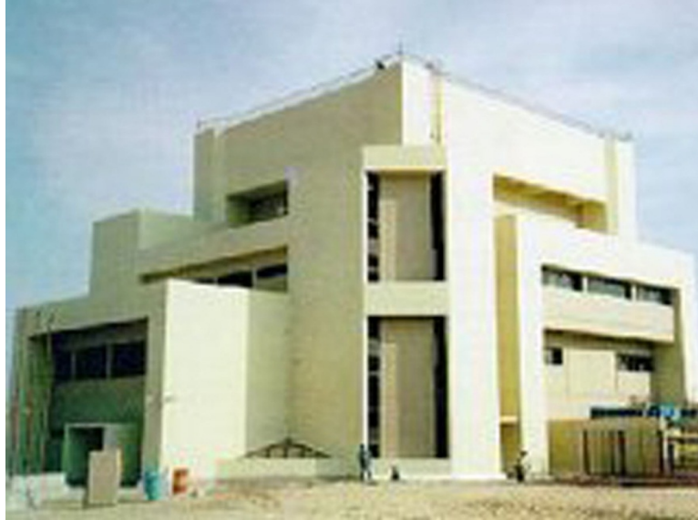
Figure 19. Exterior of the Egypt Research Reactor ETRR-2, 22 MWth research reactor at Inshass, Egypt.
