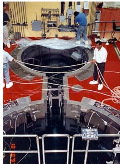
Figure 20. Interior views of the ETRR-2, open pool type 22 MWth research reactor at Inshass, Egypt.
