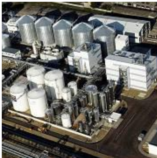
Figure 23. Neckermann biodiesel factory in Eastern Germany. DDP photograph.
