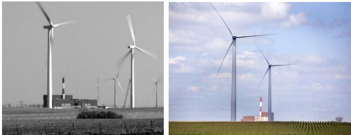
Figure 40. Symbiotic coupling of nuclear and wind technologies views during winter and summer. The two-units 2,309 MWe Boiling Water Reactors, BWRs LaSalle nuclear power plant near Marseilles, Illinois operated by Exelon Nuclear corporation and the Grand Ridge Wind Farm operated by Invenergy LLC in the adjacent farmland near Ransom in Illinois, USA. The nuclear reactor and the wind turbines are both manufactured by the General Electric (GE) Company. The GE 1.5 MW SLE wind turbines have a hub height of 80 m and are net recipients of electrical power from the grid at 5 kWe on a standby basis for its HVAC (Heating, Ventilation and Air Conditioning) system, but then become net exporters of electricity into the electrical grid under favorable wind conditions.
