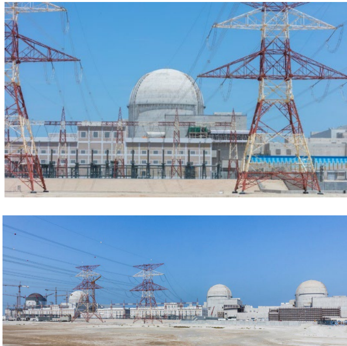
Figure 29. The Barakah four-unit South-Korean-designed APR-1400 reactors are being built at Barakah, in the Dhafrah region of Abu Dhabi, United Arab Emirates (UAE) by a consortium led by Korean Electric Power Corporation (Kepco). Construction began on the first unit in July 2012, unit 2 in May 2013, unit 3 in September 2014 and unit 4 in September 2015. The Barakah plant was developed by the Emirates Nuclear Energy Corporation (ENEC). The 1,400 MWe Unit 1 started operation in August 2020. The four units are expected to supply 25 percent of the UAE's electricity demand.
