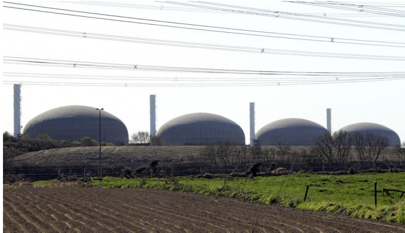
Figure 27. The Paluel four-unit nuclear power station, Northern France.
