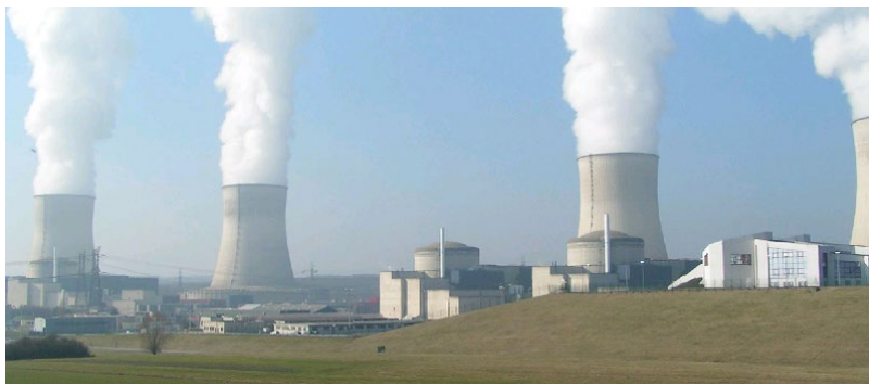
Figure 28. The Cattenom four-unit nuclear power station, and their cooling towers, France.
