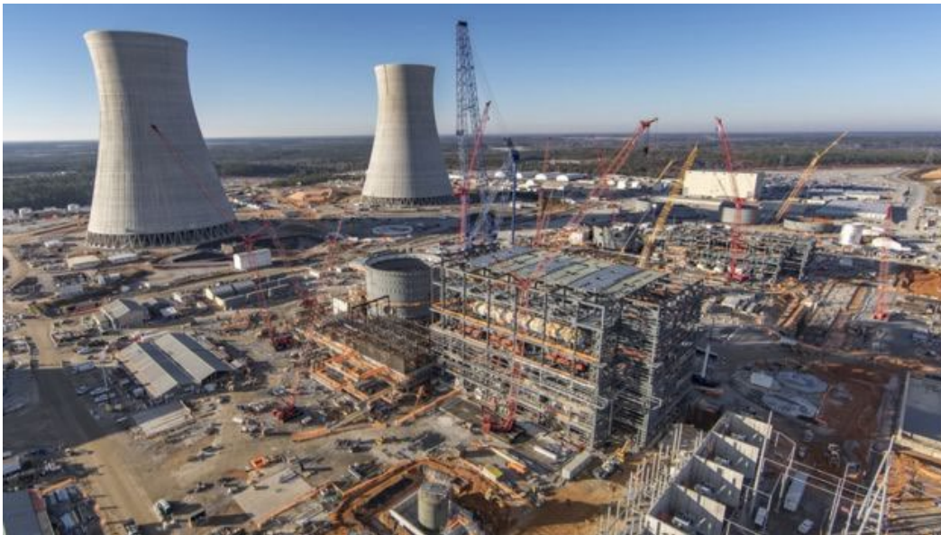
Figure 52. Cooling Towers of Vogtle plant units 3 and 4 under construction.
