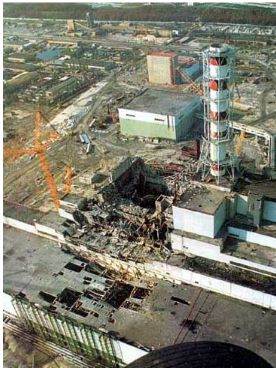
Figure 1. Damaged unit 4 of the Chernobyl plant, before being enclosed in a concrete silo.
