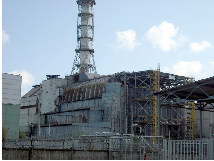
Figure 21. Chernobyl unit 4 silo under construction.
