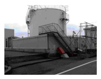
Figure 33. Earthquake-caused ground subsistence around light oil storage tank of 30,000-40,000 gallons capacity, 1979. Source: Tepco.
