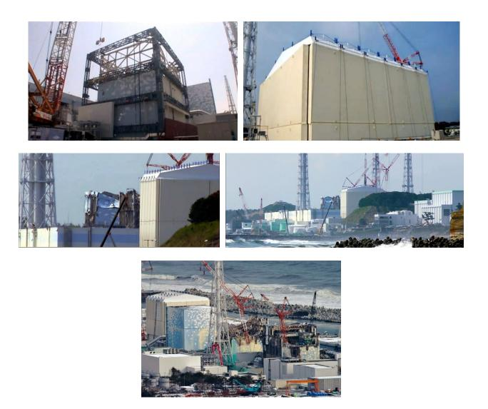
Figure 83. Cocoons encasing the damaged Fukushima reactors.
