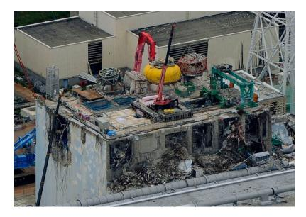
Figure 98. Debris and fuel elements removal from fuel storage pools at Fukushima.
