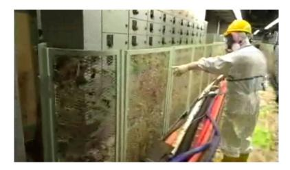
Figure 47. Tsunami water flooding of electrical switching components in basement of unit 1, May 6, 2011. Source: Tepco.
