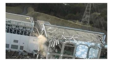
Figure 57. Fukushima Daiichi unit 4 on March 16, 17, 2011 showing steam emanating from fuel storage pool. Source: Japan Self Defense Force.
