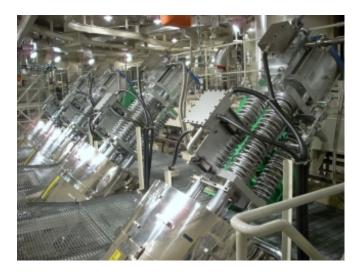
Figure 15. BWR Main Steam Isolation Valves, MSIVs. Source: Tepco.
