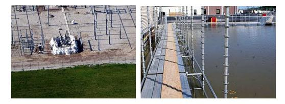
Figure 91. Circuit breaker 345 kV at transformer substation protected with sandbags and walking bridges around buildings were implemented against flooding at Fort Calhoun, Nebraska, June 13, 2011. Source: OPPD.
