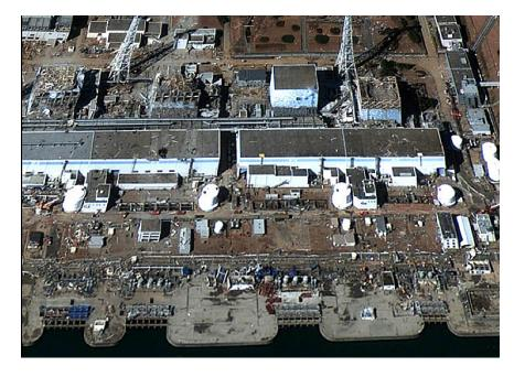
Figure 80. Aftermath of Fukushima Daiichi accident on March 18, 2011, one week after the accident. Rubble from hydrogen explosions in units 1, 3 and 4 and fire in unit 3 is spread over the site. Damage from earthquake and tsunami to the electrical systems apparent along the water front. Steam still emanating from unit 2. Source: Digital Globe.
