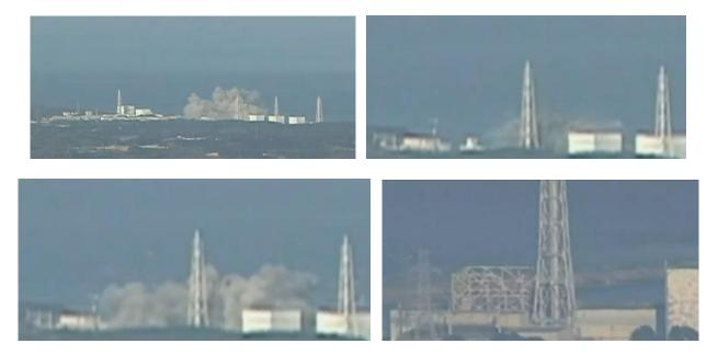
Figure 58. Fukushima Daiichi unit 1 Boiling Water Reactor, BWR nuclear power plant lateral horizontally propagating hydrogen explosion, initiated by depressurization and steam venting, sequence of events. March 12, 2011.
