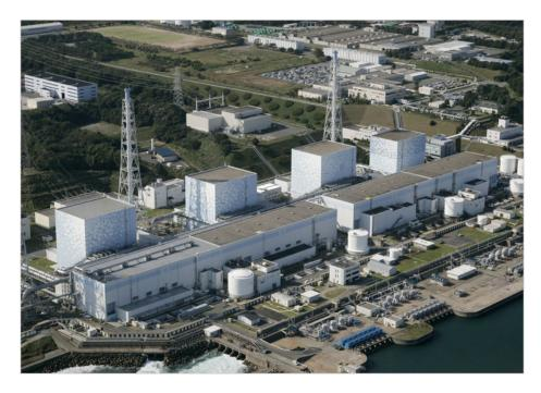
Figure 35. Fukushima Daiichi Boiling Water Reactors, BWRs nuclear Power plant, at Okumamachi, Fukushima Prefecture, Japan. The reactors are cooled with ocean water and are situated 148 miles or 238 km northeast of Tokyo. Connection to the grid shows up at the upper left side. Source: AP.
