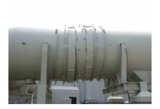
Figure 34. Earthquake-caused displacement of connecting duct to the main ventilation stack, 1979. Source: Tepco.
