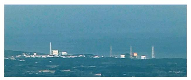
Figure 59. Lateral horizontally propagating hydrogen explosion at second chimney from the right preceded the vertical suspected steam explosion at unit 3.
