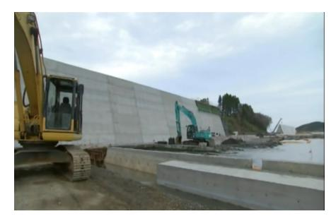
Figure 100. Concrete tsunami protection wall constructed along 400 km of the Japanese coastline.
