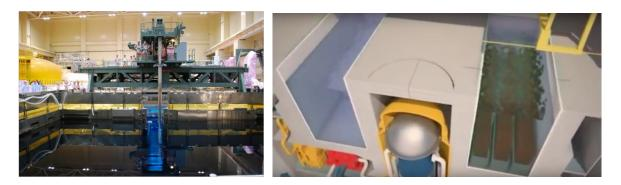
Figure 51. Refueling operation into fuel storage pool. Yellow object is the removed core dome.
