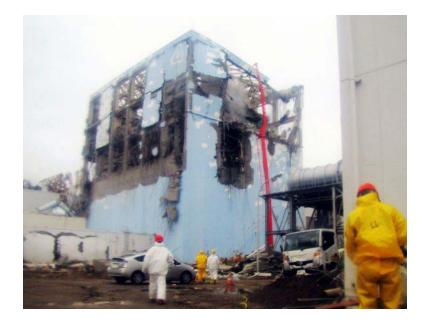
Figure 86. Damage below the fuel storage pool in unit 4 as seen from the ground on March 22, 2011. Water being pumped into the damaged spent fuel pool using a boom. Source: Tepco.
