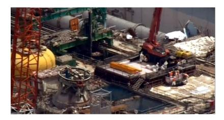
Figure 99. Extraction of fuel elements from fuel pool of unit 4.
