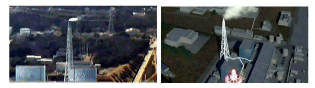
Figure 17. Venting primary containment of unit 2.
