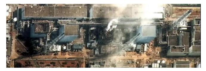
Figure 30. Remnants of a hydrogen explosion in Fukushima unit 1 (far left) exposing reactor loading deck and burying it under concrete rubble. Fire and a hydrogen explosion associated with steam depressurization and fuel damage occurred in unit 3. Fire starting at side of building in unit 4 may have originated from hydrogen generated in unit 3 that was piped into the shutdown unit 4, on March 15, 2001. Photo: DigitalGlobe.
