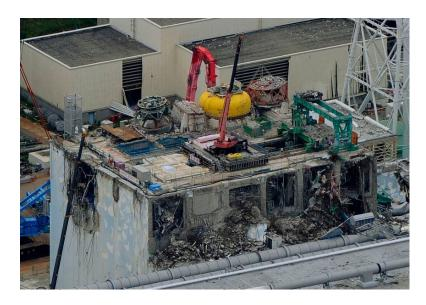
Figure 95. Debris removal at Fukushima unit 2.
