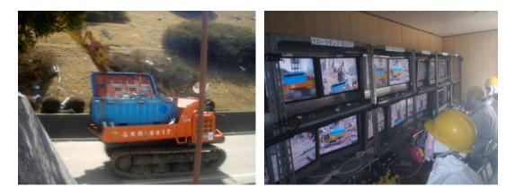
Figure 84. Removal of debris using remote control equipment and autonomous transporters. A useful design feature at the Fukushima site is an emergency command control center in an earthquake proof bunker with power supplies, radiation shielding thick walls, communication gear, food and water supplies and two air filtration systems. Source: Tepco.
