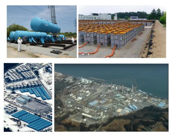
Figure 87. Storage tanks for sludge resulting from the water decontamination process and coolant storage tanks. Contaminants are removed except for tritium, which decays with a 12.3 year shalf-life. Source: Tepco, DPA.
