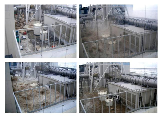
Figure 12. Fukushima Daiichi Tsunami water ingress and egress, drowning plant components at the base of the ventilation stack system, March 11, 2011. Source: Tepco.
