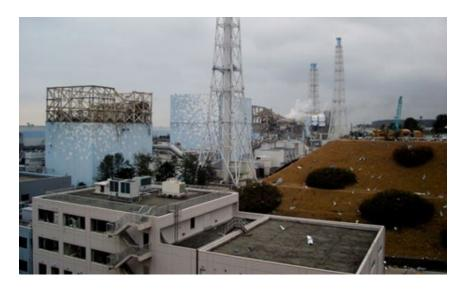
Figure 53. Damage to the upper structure of the Fukushima Daiichi unit 1, and undamaged structure of unit 2. Source: Tepco.
