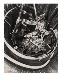
Figure 64. Damaged core resulting from steam explosion caused by a criticality accident in the military Small Low power reactor experiment SL-1 BWR. A worker inadvertently yanked out a control rod beyond the set limit during a maintenance procedure. The core became supercritical, boiled off the steam causing a steam explosion. The drying of the moderator stopped the fission reaction, even though the decay heat generation would have persisted for a while.
