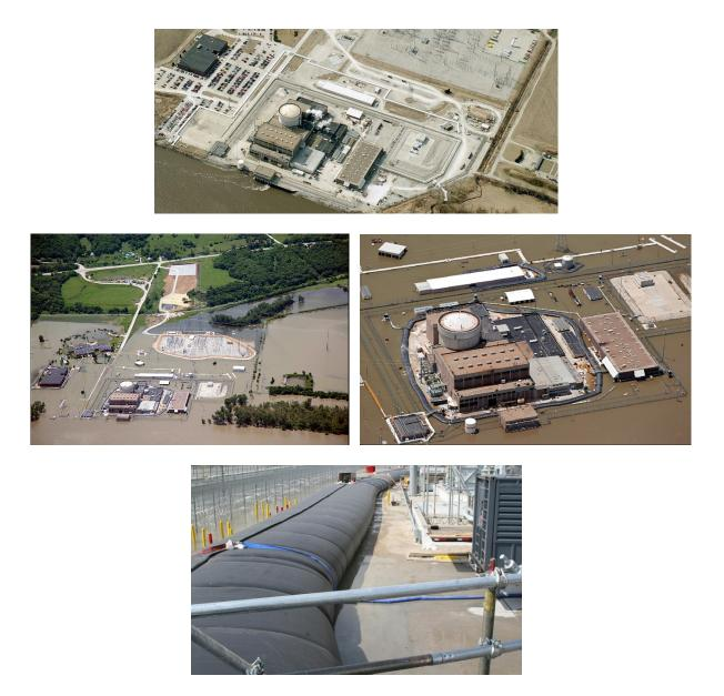
Figure 89. Fort Calhoun station, Blaine, Nebraska, 19 miles north of Omaha on the Missouri River is protected against flooding by a 2,000-ft long Aqua Dam berm from releases from the Gavins Point Dam, June 10, 2011. The berm raises the protection 6 ft above the 1,004 ft river level to the 1,010 ft Mean Sea Level, MSL. Source: OPPD.
