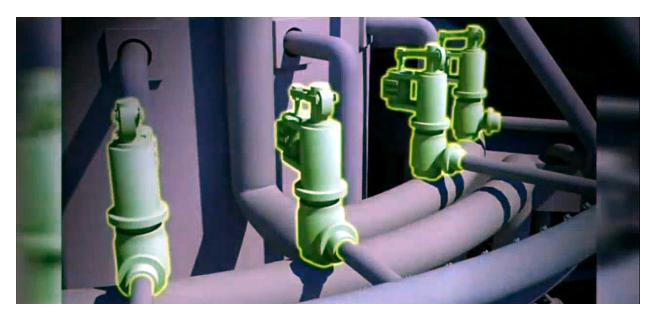
Figure 19. Bank of 8 safety relief valves of the primary containment failed to operate to vent the hydrogen and steam pressure from the containment.
