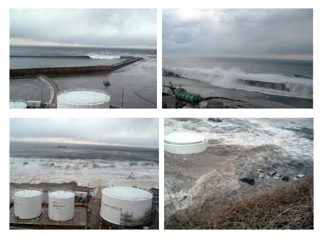
Figure 7 The tsunami wave more than 14 m (46 ft) high that originated 125 miles (200 kms) to the East, impinging on the 6 m protective wall and drowning the Fukushima Daiichi nuclear power plant site, March 11, 2011, Japan. According to the plant design, the maximum probable height of a tsunami at Fukushima was at just 5.7 meters compared with the actual 14 m. The breakwater wall offered protection against typhoons, but was breached by the tsunami. Source: Tepco.
