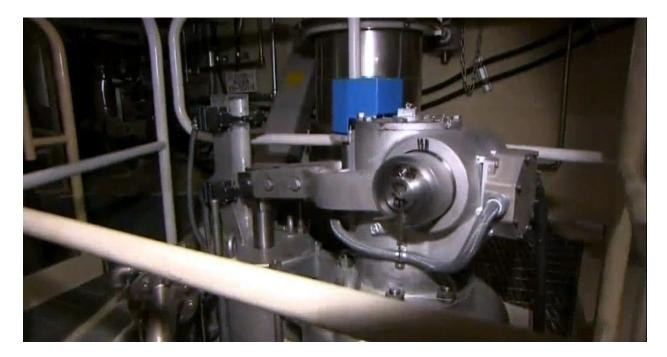
Figure 27. Safety relief valve picture.
