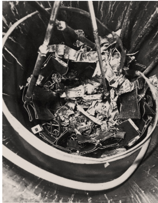
Figure 5. Top view of the damaged SL-1 core.
