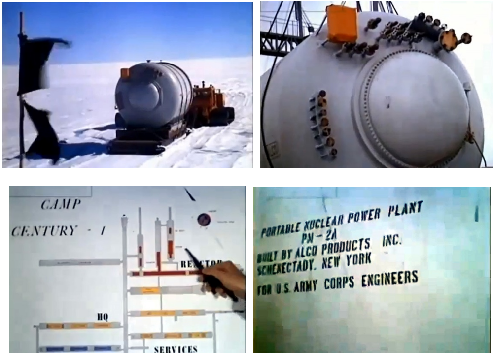
Figure 6. USA Army's Camp Century-1, Greenland, Denmark Portable Nuclear Power plant PM-2A, pressure vessel. Source: USA Army.
