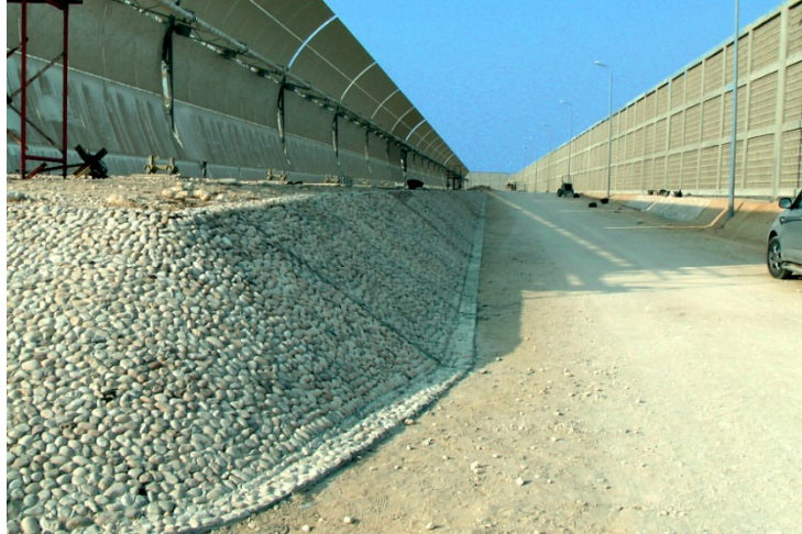
Figure 3. Gravel substrate and surrounding rigid wall for dust and wind suppression at Al Kuraymat, Egypt [16].
