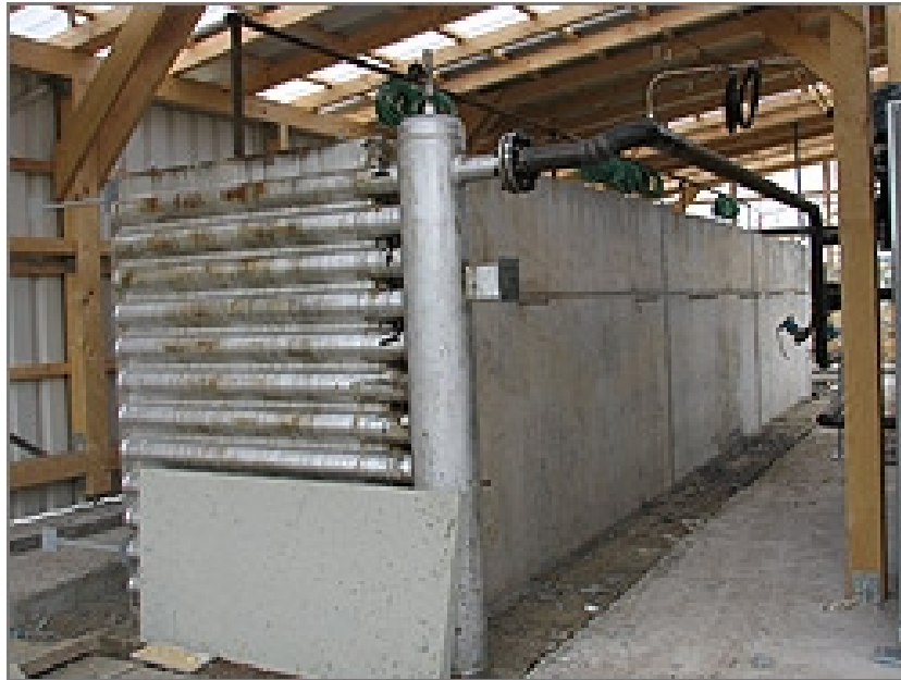
Figure 2. Concrete thermal energy storage unit.
