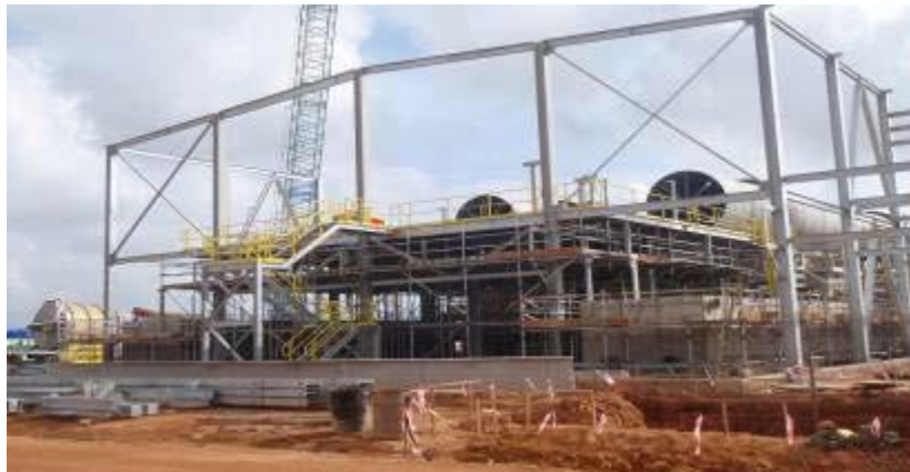
Figure 24. Primary leaching building.
