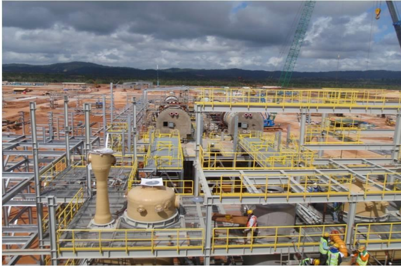
Figure 37. Cracking or Rotary Kiln at Lynas Advanced Materials Plant (LAMP) Rare earths refinery operated by Lynas Corporation at the Gebeng Industrial Zone, Pahang, Malaysia. Source: Lynas Corporation.
